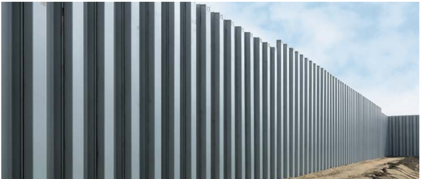
Coated and sealed retaining wall, Essen
